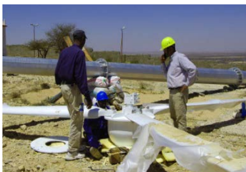
SECCCO Energy, Qardho Hospital Solar Panels
