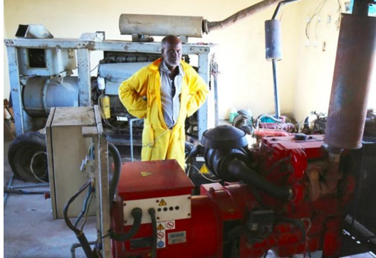
A Beder Electric Co. technician stands between a diesel generator and a generator run by a wind turbine in Ainabo.
